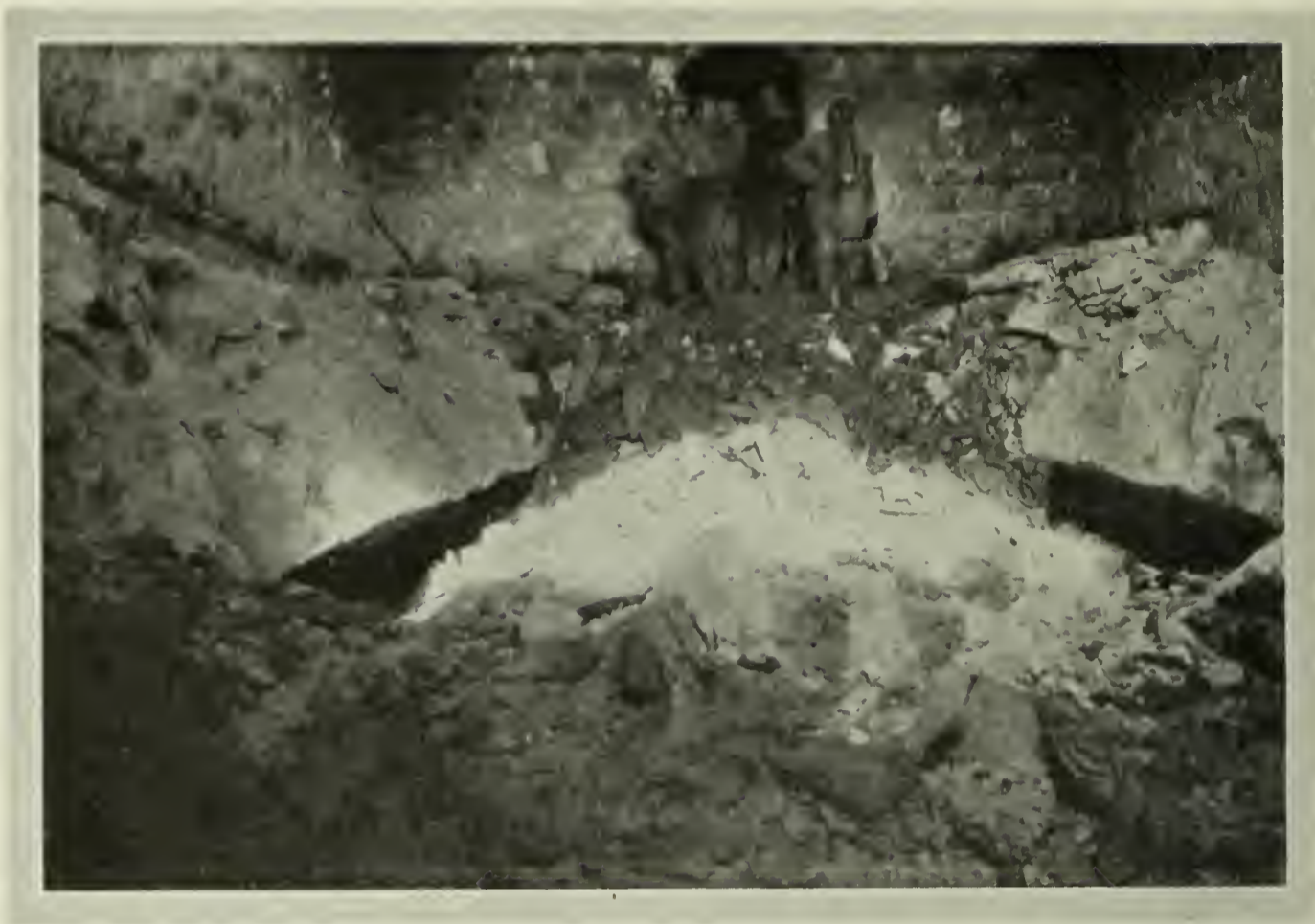
WRECKED CASEMATE OF DOUAUMONT FORT.
