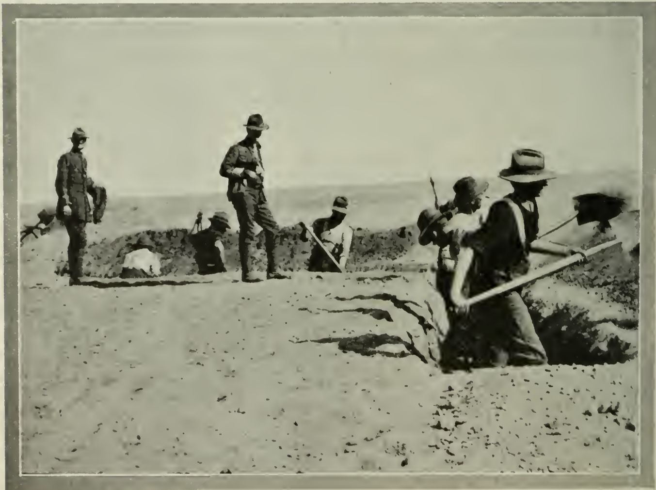
TRENCH-DIGGING IN THE DESERT.
