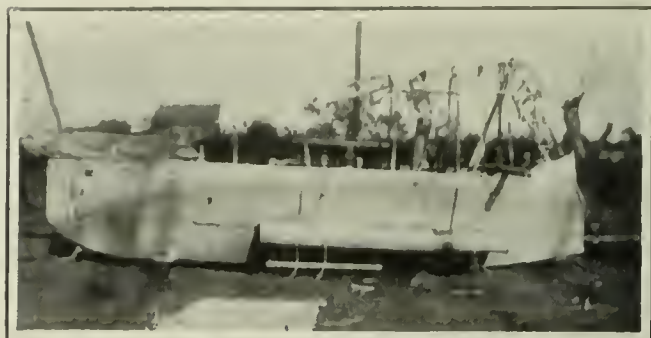
THE PORT SIDE GONDOLA OF L 33.
