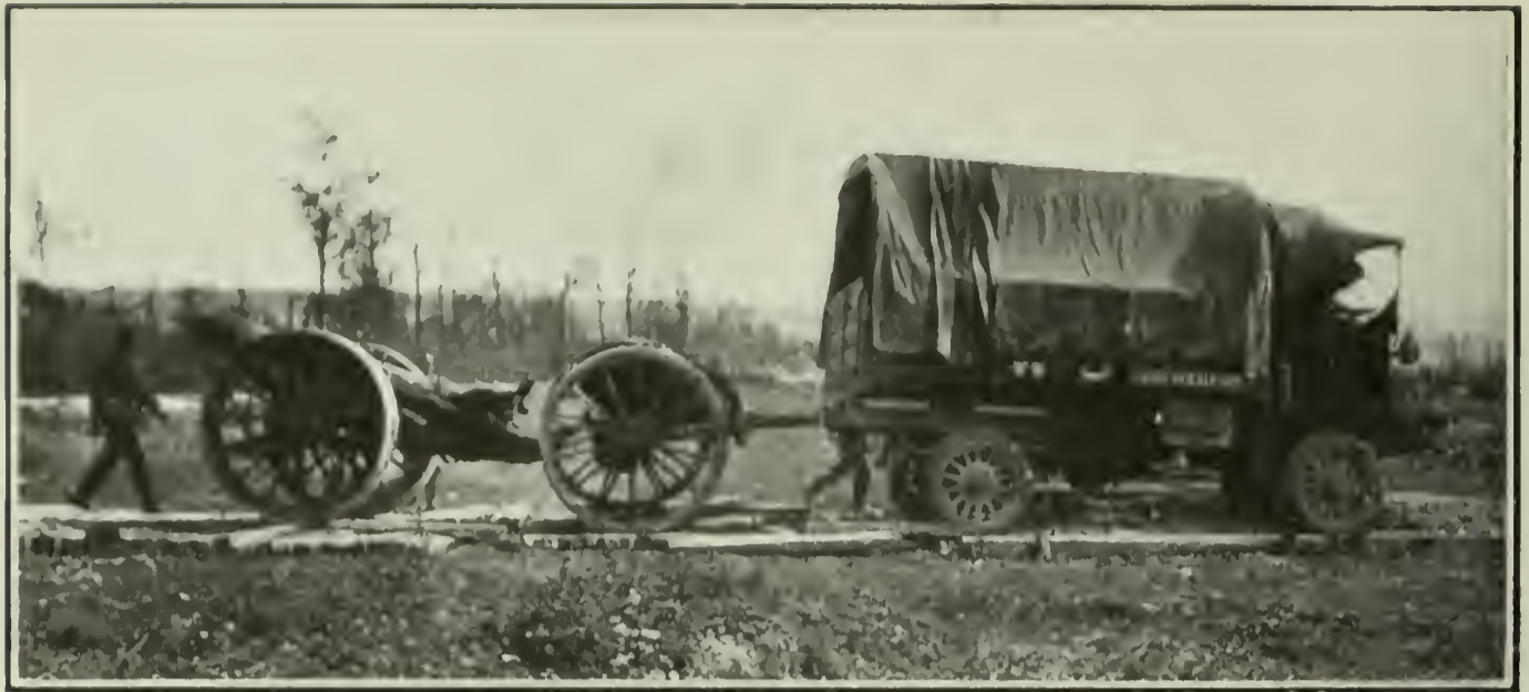
A MOTOR LORRY AS TRACTOR. Bringing up a howitzer on an improvised track.
