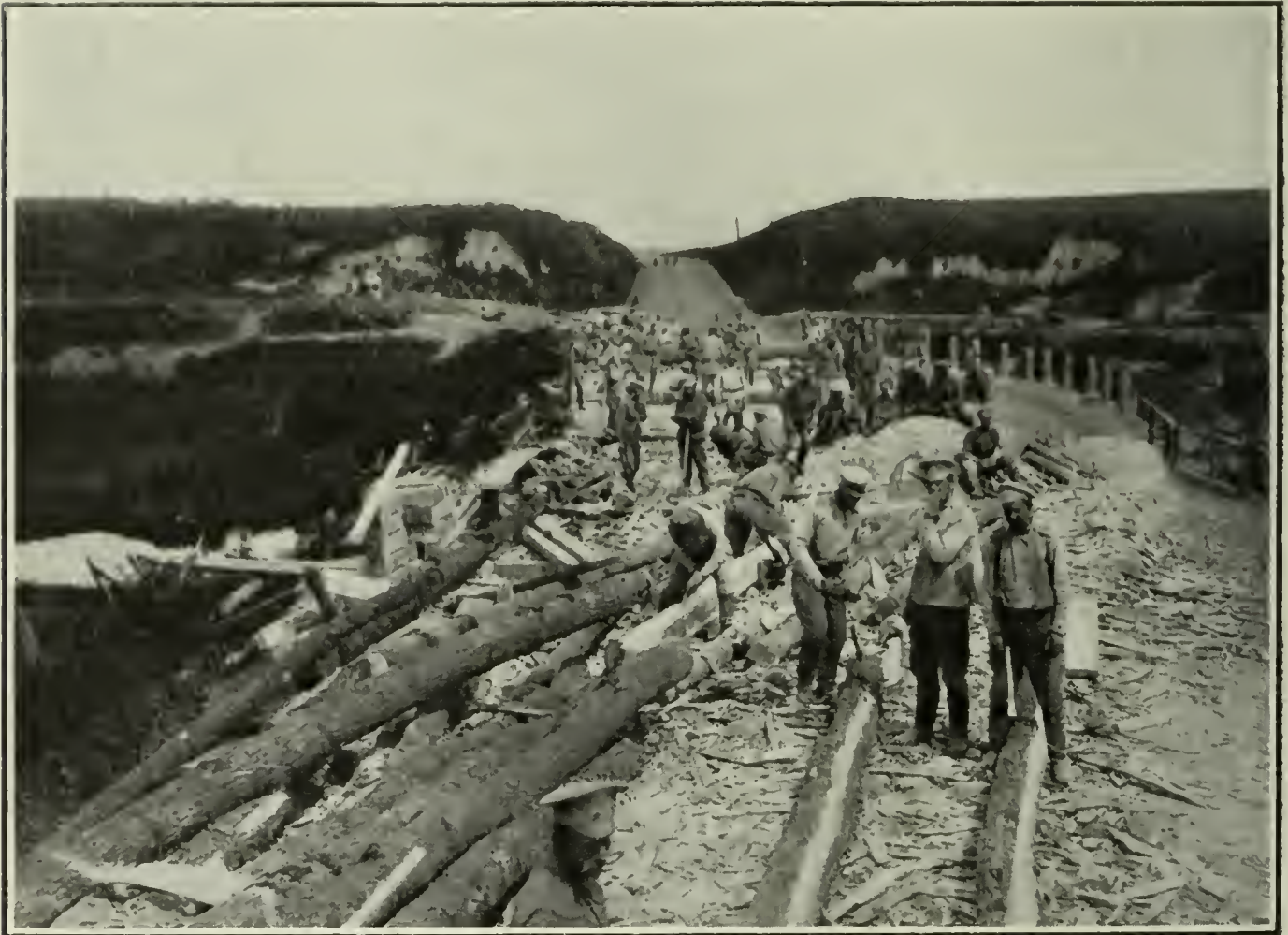
REPAIRING A BRIDGE BLOWN UP BY THE AUSTRIANS.
