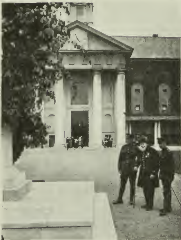
THE ENTRANCE TO THE HOSPITAL.
