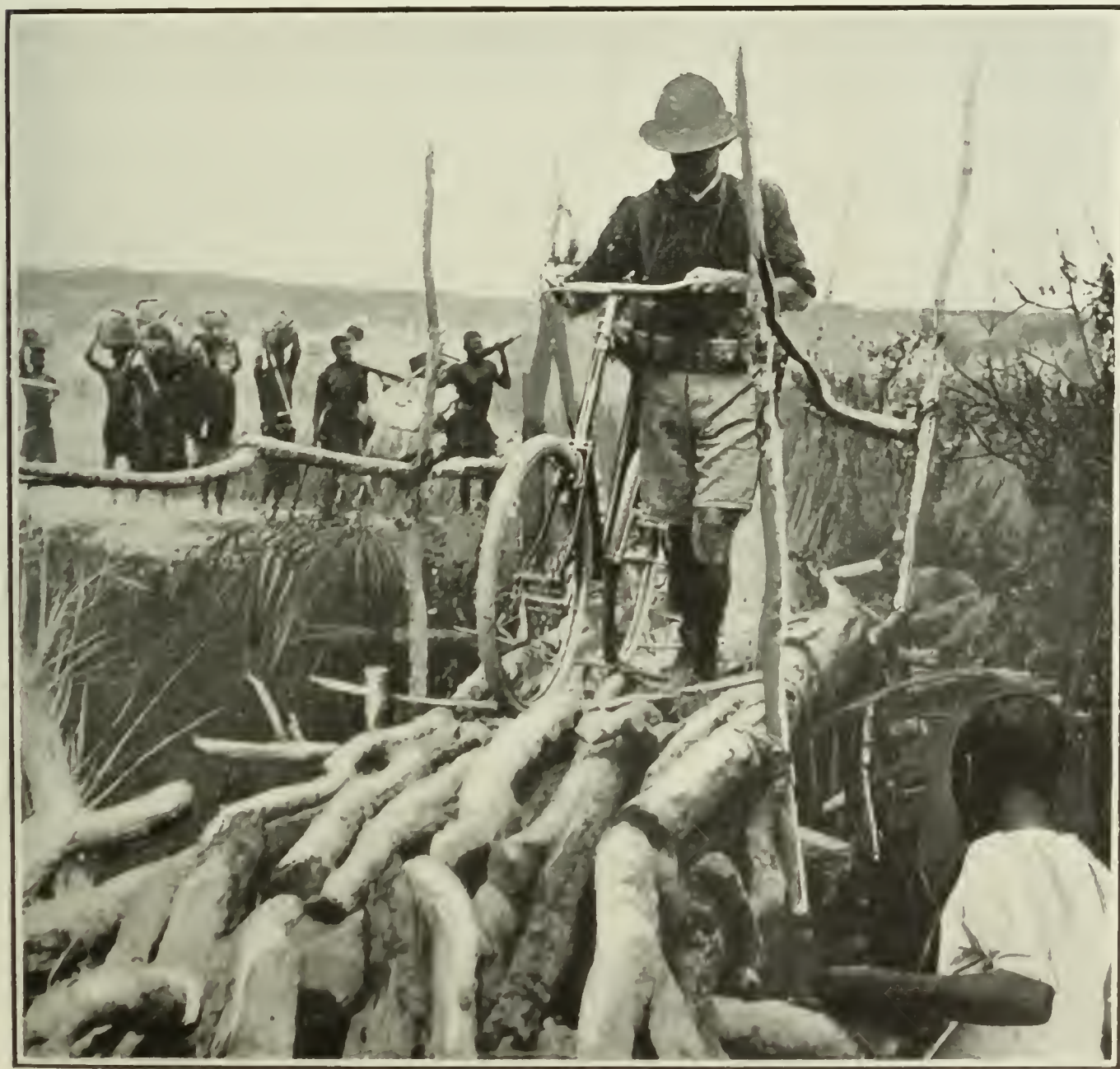
DISPATCH-RIDER CROSSING AN IMPROVISED BRIDGE.
