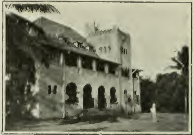
GOVERNMENT BUILDING, DAR-ES-SALAAM.
